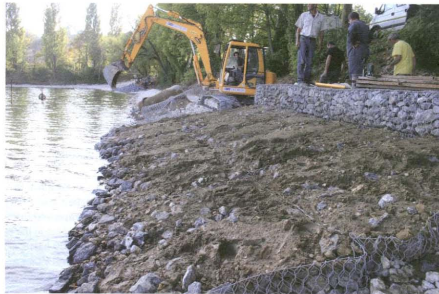
Photo 5 Pose des gabions et matelas de gabions Laying gabions and gabion mattresses
